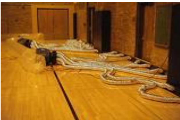
The photo to the left demonstrates the previous example. Two high velocity air movers are forcing the, 100 deg. 8% RH at 31gpp. (grains per pound) air under the floor. The floor is still very accessible to walk on and monitor progress. Air intake should be monitored and documented daily to assure that the gpp is under 40 to assure the floor is drying properly. This can be achieved by using any standard issue thermal hygrometer and a psychrometric calculator.
