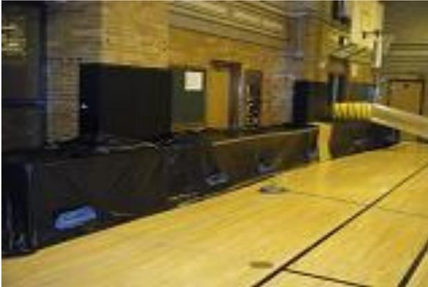
This photo shows the opposite side set up under negative air pressure which creates a vacuum under the floor assuring that the desiccant air reaches the entire affected area of the floor. Each of these air movers should be monitored and documented daily to insure that the process is working. Each day should show a slight decrease in the gpp daily if the air is evaporating moisture properly.
