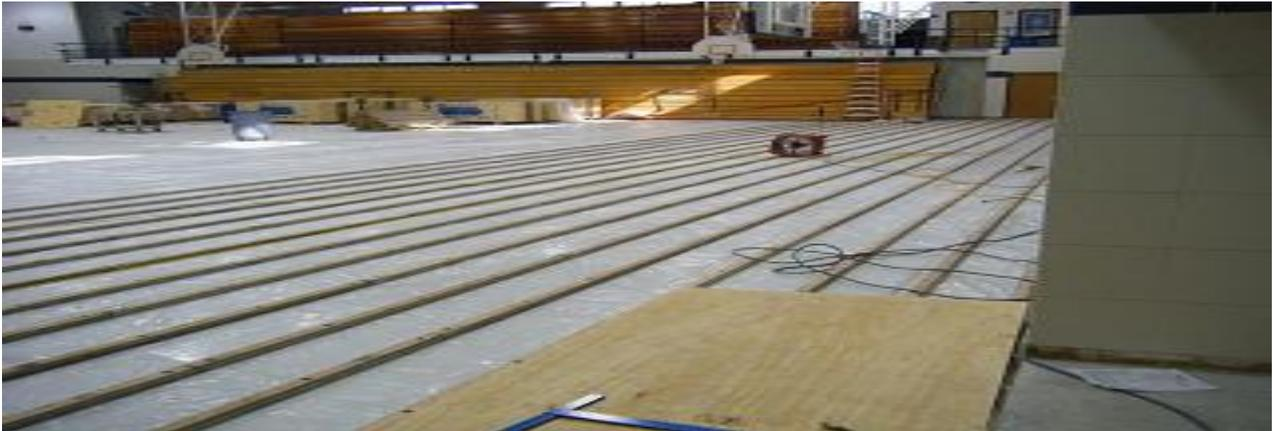
Above is a standard floating gymnasium floor. The technique I have found after many attempts to be the fastest and most effective way to dry gym floors by utilizing the channels created during the construction of the floor. The channels run from one end of the floor to the other.
